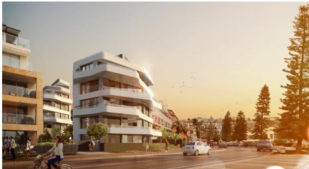
Building front view
