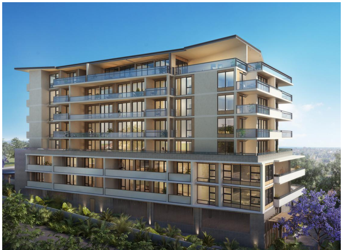
Building side view
