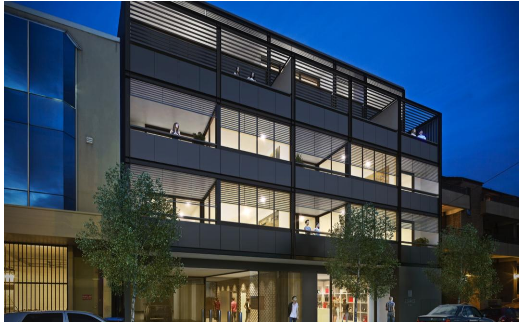
Building front view
